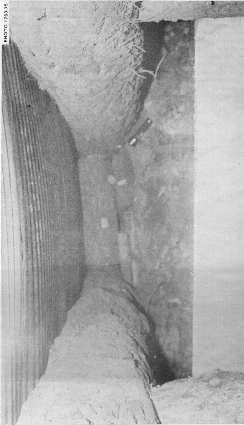
Fig. 7.5. Parts of the roof-boards and two roof-logs, each with its supporting column-log, of the large Log-Covered Trench Shelter built in Colorado in 1972. This 45-occupant Colorado shelter had a different roof design than that of the 50-occupant Alabama shelter; its 22-ft roof logs were of larger diameters, were spaced 2\frac{1}{2} to 4 ft apart, and were covered with 2-in. boards or heavy corrugated iron roofing laid parallel to the length of the bulldozed trench. Each of the thick 22-ft roof logs was supported in its center by a column-log. Each column-log was notched with a flat V on top, as illustrated by the tops of the two column-logs shown in this picture.
